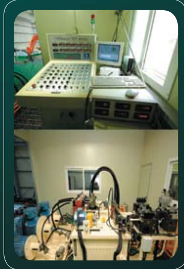
Control console with monitoring panel. Power pack to replicate actual situation.
