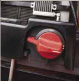
Battery cut-off switch
