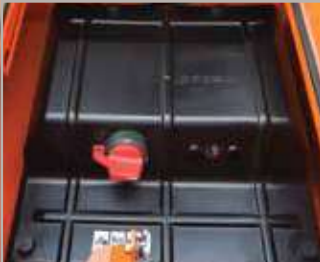
Battery cut-off switch
